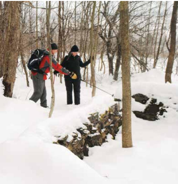
▲ Dennis Stier of Southampton and Peter and Carol Harris of Owen Sound examine features of the Mystery Cabin foundation. It is unknown who began this structure or when, but it remains uncompleted.
